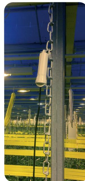
The large water content in plants and fruits is the primary factor contributing to the weakening of the radio signal if sensors or the base station are positioned too low. The sensor has an extended wire to a transmitter - position the transmitter (white body approximately one foot or 30 centimeters above the expected maximum height of the plants).
