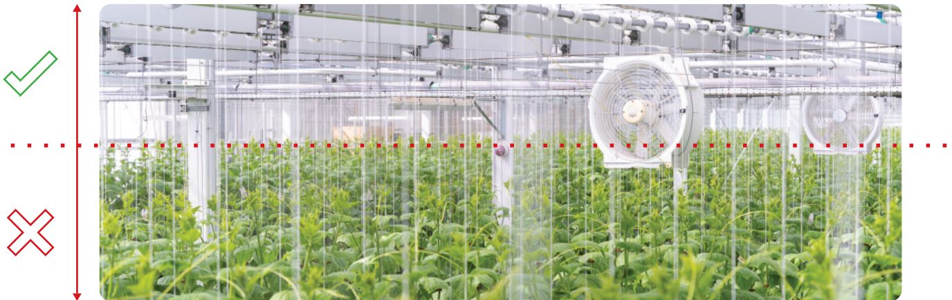
Example of the Base station installed above the tomato plants in the greenhouse.
