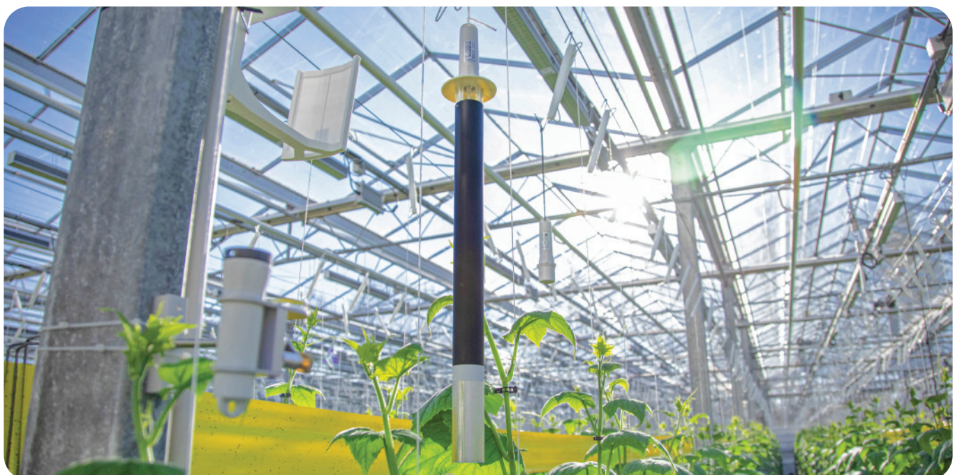
Example of PAR, T/RH with a Radiation shield, and CO 2 sensors installed in the greenhouse to monitor ambient conditions
